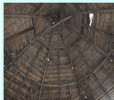
Casa Miraflores roof riddled with holes, especially in the upper parts © TReeS
